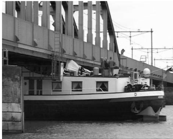
Fig. 7. Collision with the bridge on Elbe river [4]
