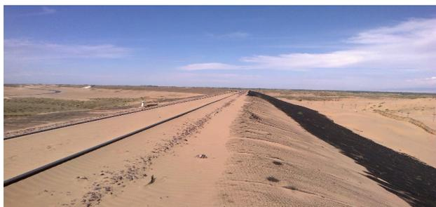
Fig. 1. Sandy drift of a railway track near the station Altynkol (Kazakhstan)
